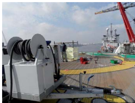
Image 3: Removal of the old paint
