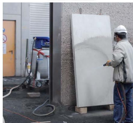
Image 9: Blasting test of a concrete element
