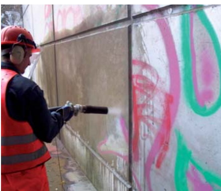
Image 7: Removal of graffiti with torbo
