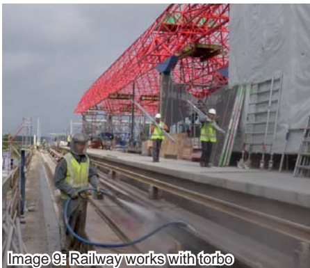
Image 9: Railway works with torbo
