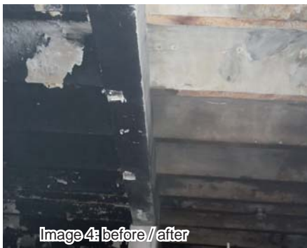
Image 6: after the cleaning with torbo
